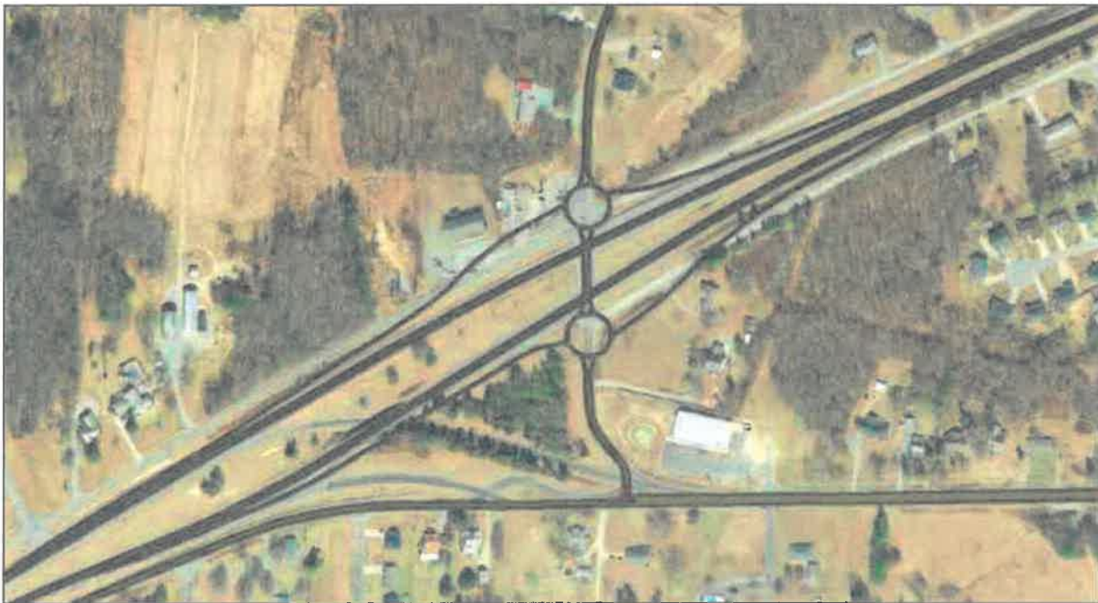
Planned Improvements associated with SPOT ID: H170582 at the I-85 Business Interchange at Kanoy Road [Source: NCDOT's Travel Time Summary (TTS) Report for SPOT ID: H170582]
